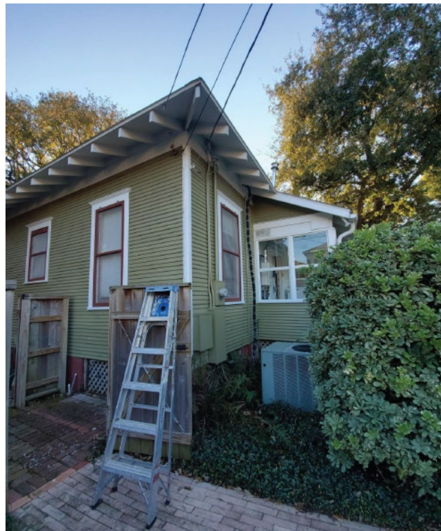
Figure 8- East Side Rear Corner
